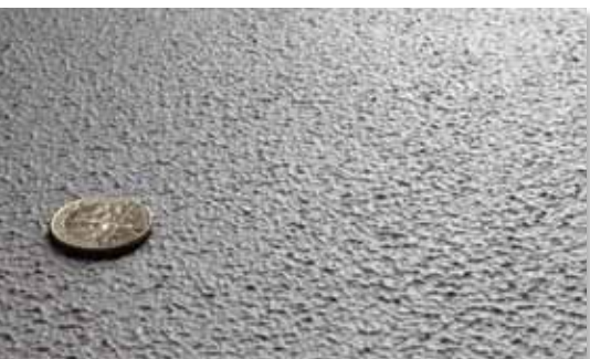
..... KiwiGrip was the only paint that did not use a nonskid compound. Its no-slip texture comes from a unique roller sleeve.
